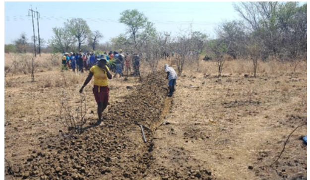
Community members at the Mzinyathi borehole during drilling (top) and digging trenches to lay pipelines for connecting Mzinyathi buildings to the water tank
